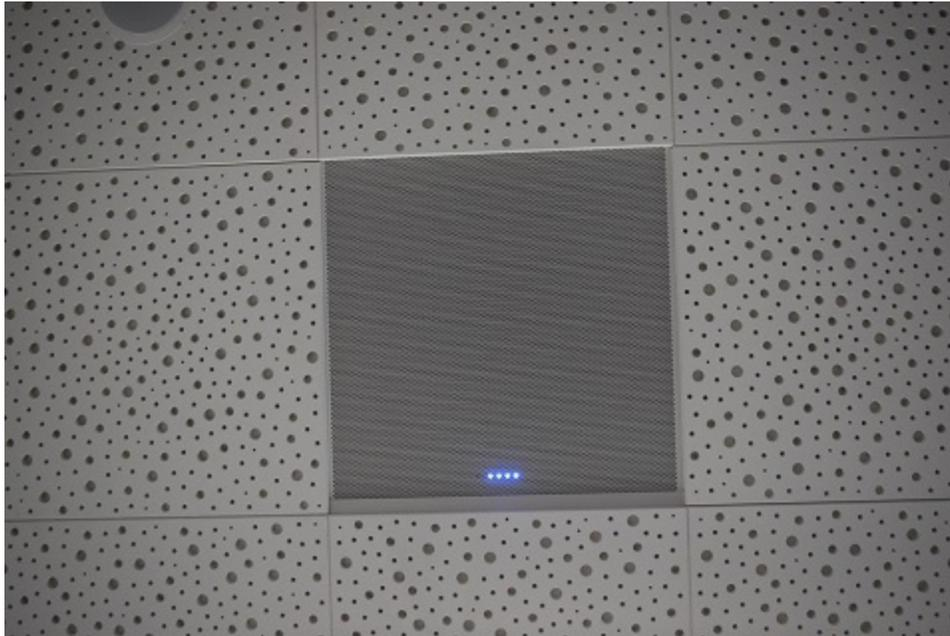
The BMA 360 with Voice Lift and Camera Tracking technology is the world's most technologically advanced beamforming microphone array ceiling tile
